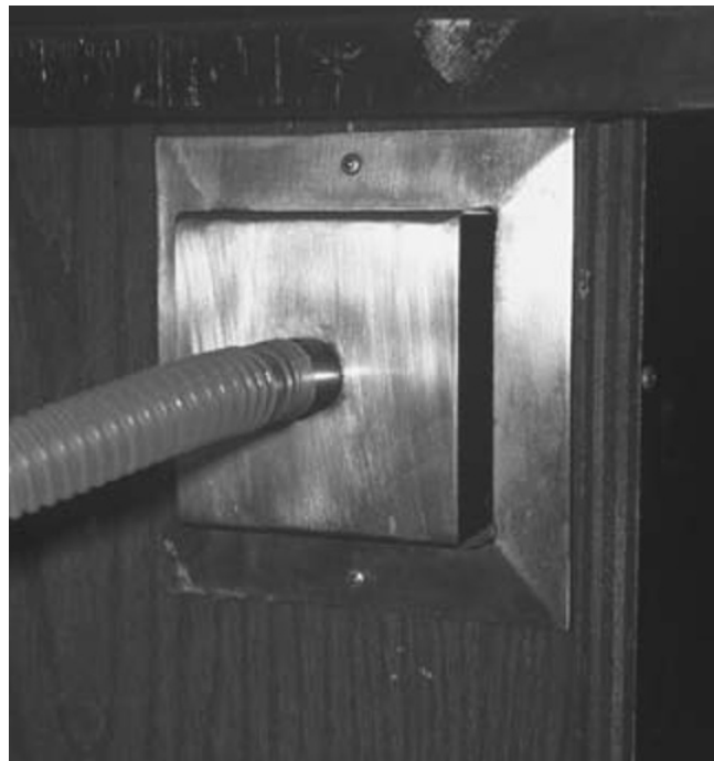
Fig. 17.64. Corrugated tubing from the pop-off valve of a circle breathing system attached to a high-volume, low-pressure scavenging system (an active duct system). Air is constantly entrained on each side of the stainless-steel plate, whereas waste gas from the breathing system enters the scavenging system through the corrugated tubing.
