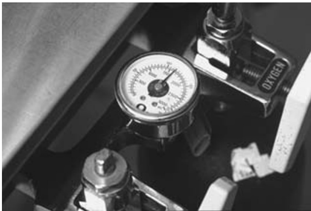
Fig. 17.68. Oxygen cylinder with the pressure gauge reading at 1700 psi after 15 min with the cylinder valve open. If the cylinder pressure was 2000 psi at the start of the test and the flowmeters were off, a significant leak is present and should be corrected before the anesthesia machine is used with a patient.
