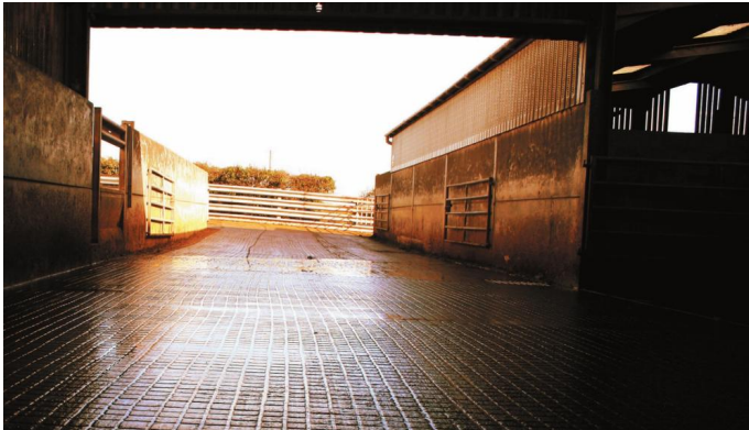
Grooved concrete provides a non-slip floor.
